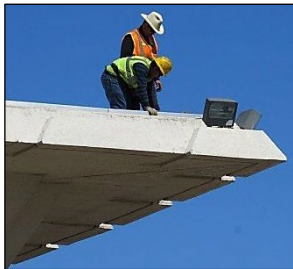
Up on the Library roof in 2016 for repairs. (Muskogee Phoenix photo)
