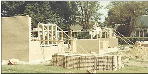
Library under construction, 1967-68. (Library Photo)
