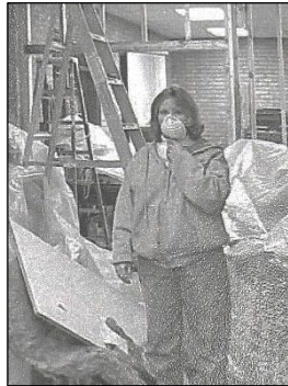
Ghormley wasn't wearing a Halloween costume in October 2002, only necessary protection during the Library's renovation. The Library closed to the public November 1 to complete the construction. (Library photo)
