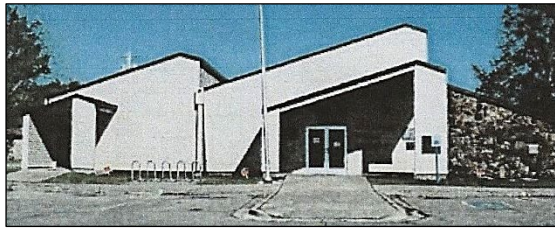
This picture illustrates the completed Phase II Meeting Room on the building's north side. (Library photo).
