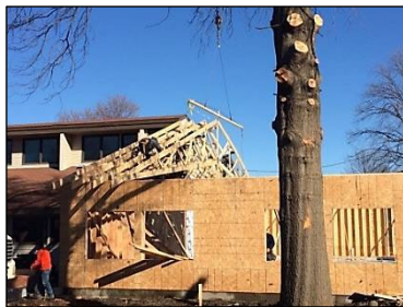
Construction underway on the Children's Wing in 2017. (Library Photo)
