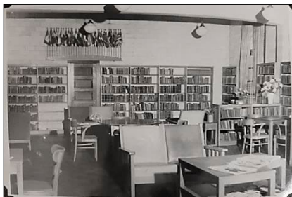
Main Room of the Wheatley Branch Library. (Library Photo)
