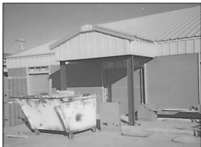
The new west front entrance under construction in December 2001. (Library photo)
