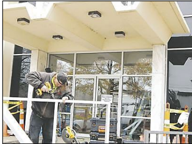
MPL front door repair, 2014. (Muskogee Phoenix photo)
