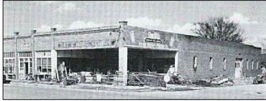
The Sellers Building, (aka Comfort Building) on the southwest corner of Williams and Division Streets before it was destroyed by fire. Westville's Utility Building currently inhabits the location. This Building served as the home for the Westville Community Library from 1960-1968. (Library photo)
