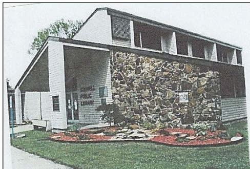
Energy-saving renovations in 2004 to helped reduce utility costs. (Stilwell Democrat-Journal)
