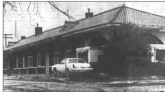
The Depot awaits renovation. The City Commissioners voted to award the contract for the renovation January 9, 1984. (Sequoyah County Times)
