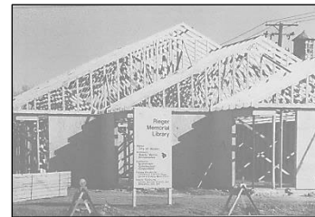
The Rieger Memorial Library in Haskell under construction, 1984. (Library photo)
