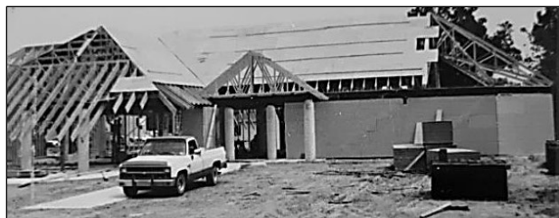
The construction of the new Library's front entrance, 1984. (Library photo)
