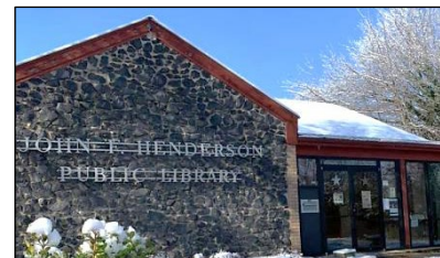
The John F. Henderson's remodeled handicapped accessible entry, circa 1988-89. (Library photo)
