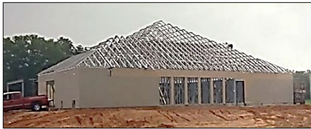
Library walls were up ready for the roof, 2004. (Library photo)
