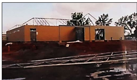
The Library's walls were up and so was the excessive moisture at the building site. (Library photo)
